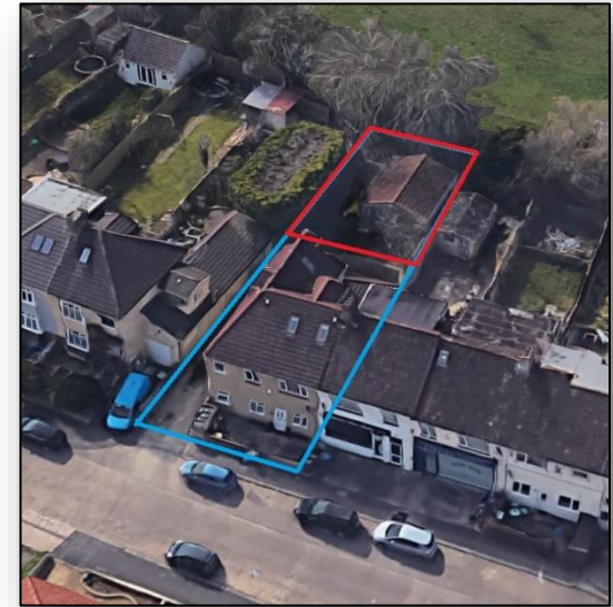
1 Ariel View showing site
